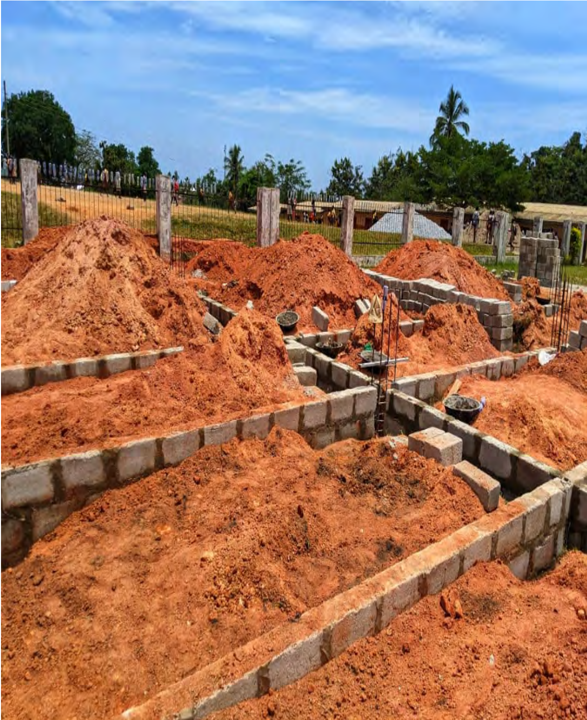
Final Block Work Level
